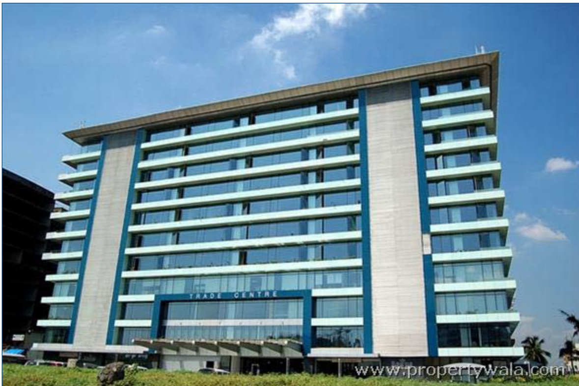
The new SCHNABEL office in the Bandra Kurla Complex, Mumbai
